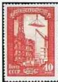
Building under Construction A990
