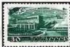
Farkhatz Hydroelectric Station A709
