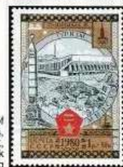
Metro Bridge, Dnieper River, Kiev — SP29f
